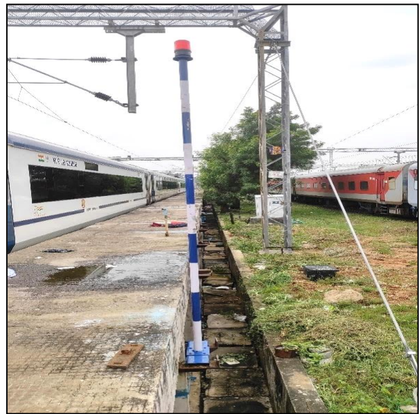
Signal pole installed on west side of pit line No. 3
